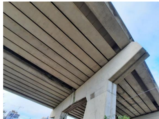
Plate 2: Underside of the A4234 Flyway
